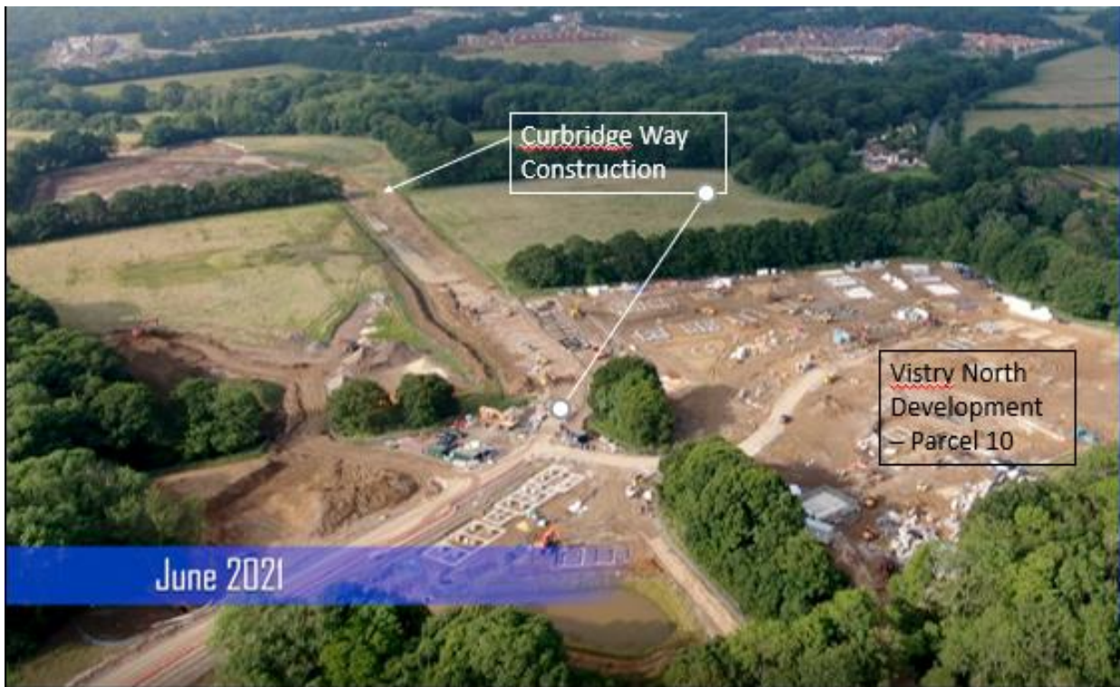
Plate 7: Curbridge Way – View South @ 30 th June 2021
