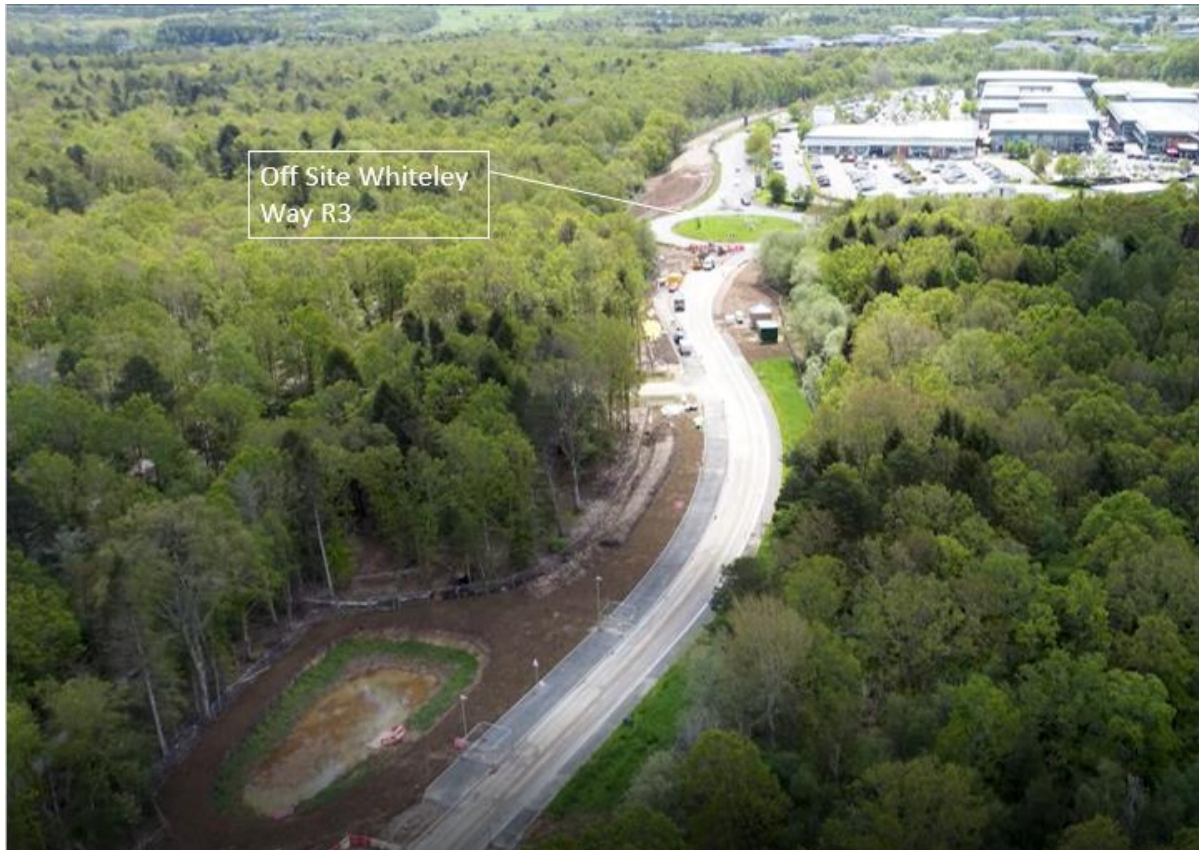
PLATE 11: View of Embankment Works from R3 looking South @ 26 May 2021
