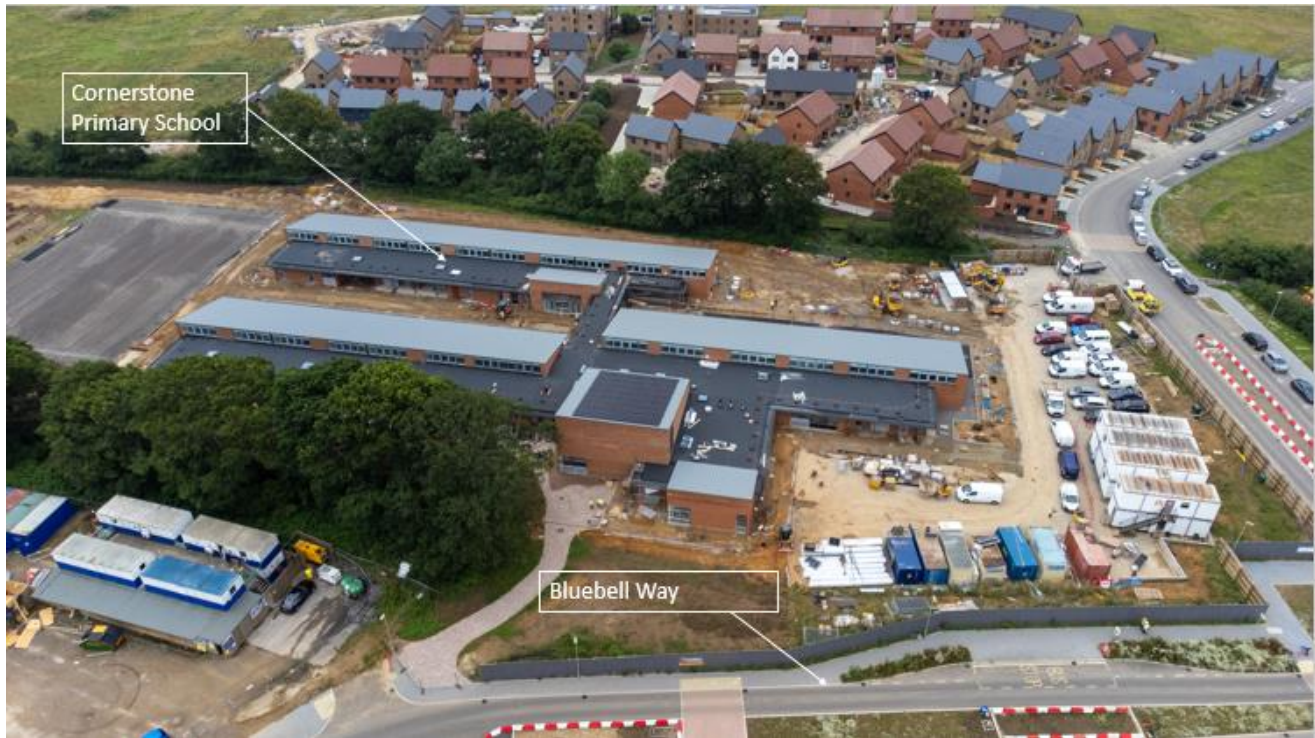
Plate 10: View South Cornerstone Primary School @ 30 th June 2021.
